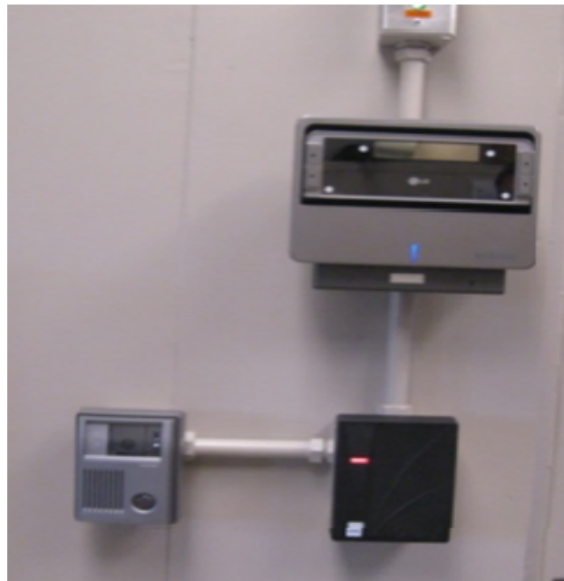
Figure 4-4 Card reader with associated iris scan biometric device
