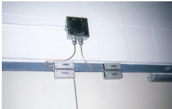
Figure 4-5 Triple-biased BMS sensor on double doors
